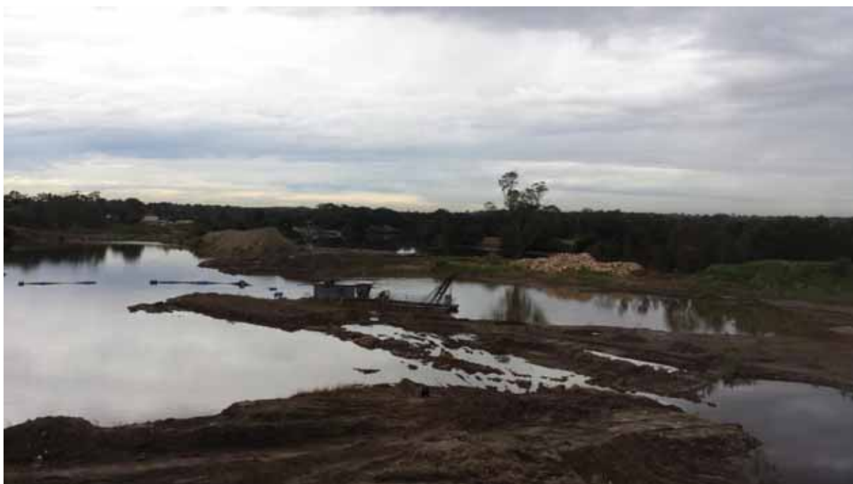
Photograph 4.1 Site condition – 29 May 2015
